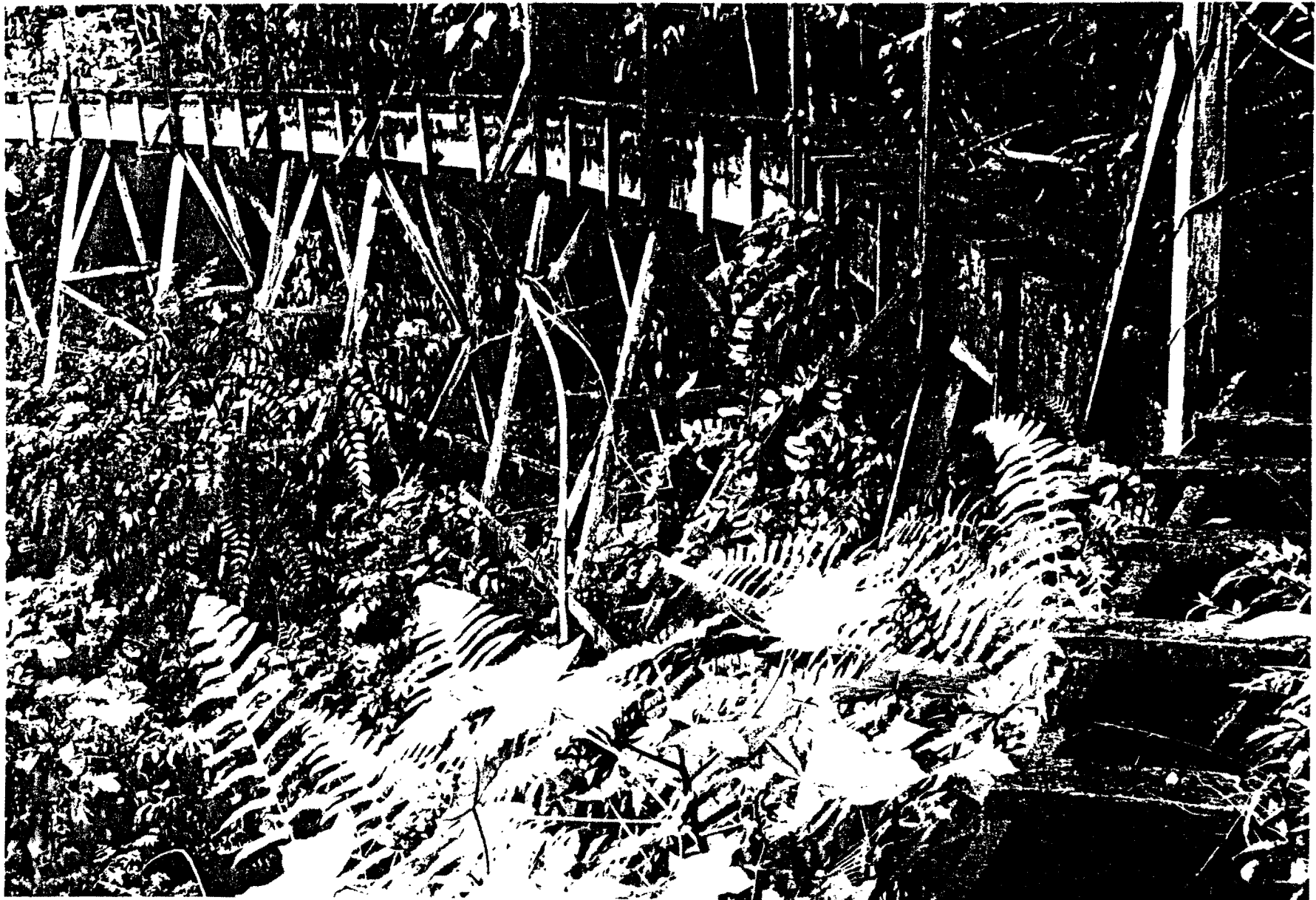
Figure 1.18 Recent Photo of Flume and Ditch Diversion System Constructed in the Upper Maunawili Valley in the Early 1900s (Photo by William Stifel)
